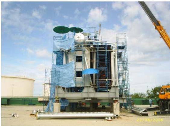
The raised position of the skids is to allow a low loader to drive under the skids to load them and carry the assembled skid to the jetty
