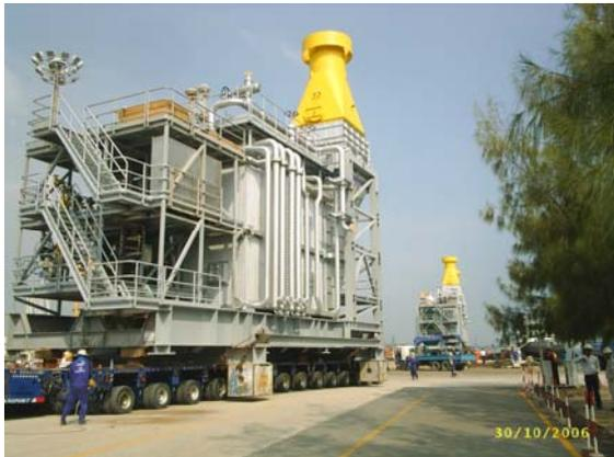
Eventually the boilers were ready for transport and were taken by low loader the 200 meters to the jetty where they were loaded out onto the barge.
