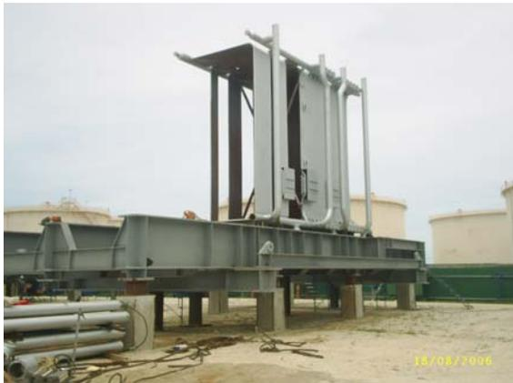
The skid base frame was designed by Naval Architects for installation on the vessel. The skid was surveyed for flatness before assembly and the unit was jacked so that the levels were retained during erection and after installation on the vessel
