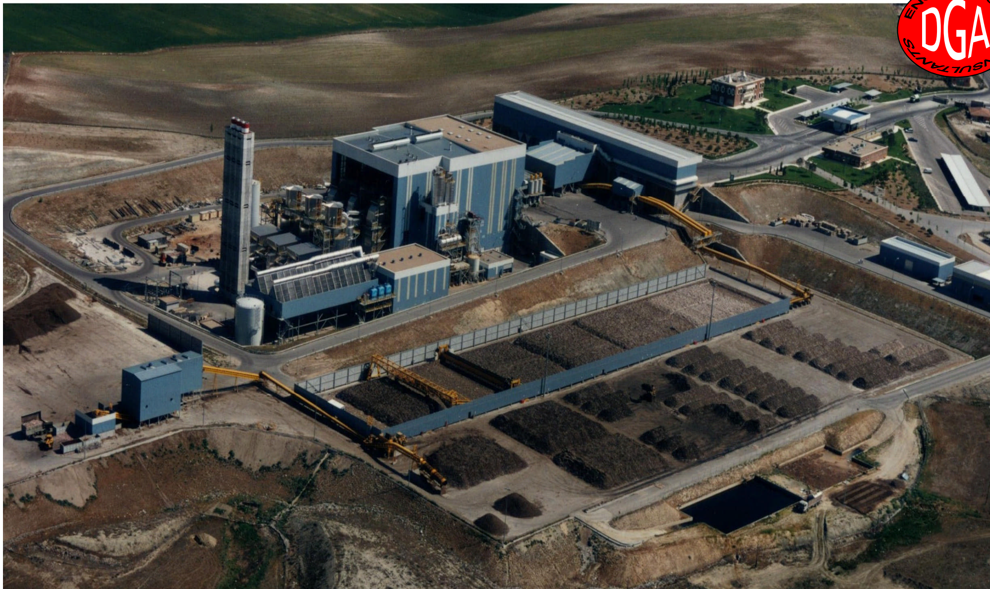
This picture shows an open composting plant producing compost from Municipal Solid Waste in Madrid, Spain not long after the plant was constructed (c 1998). The plant operates in conjunction with the 30 MWe coarse RDF fired Waste to Energy plant. The compost plant is rated for 400 tn/day of organic waste. The aeration floor uses a fixed turning machine (centre picture) operating on rails. This is supplemented by a mobile windrow machine
